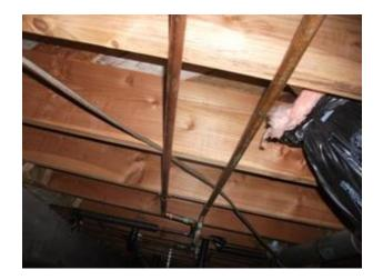
Repair: One or more joists are damaged due to non-standard or substandard notching and/or hole boring. Standard building practices specify the following limitations for notching and boring joists:
