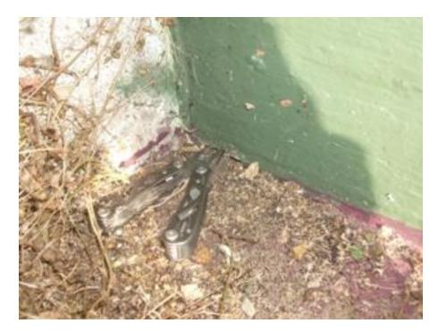
Maintain: The back deck posts need to be away from soil contact and vegetation. Even treated materials will decay over time.
