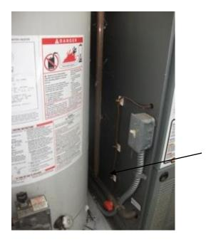
Repair: There are no seismic straps on the water heater. These are needed to keep the heater in place in a seismic event. One strap high and one strap low. I recommend someone qualified install seismic straps as required.
