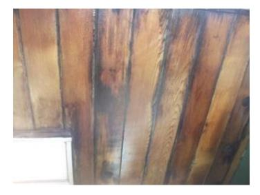
Repair: The southeast soffit has come loose. I could slightly see inside and there were two wasp nests present. They did not appear to be active. I recommend re-fastening the soffit so no insects can enter and nest.
