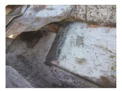
Maintain: Gutters are restricted in some areas around the roof. These need to be cleaned now and often to prevent pooling water on the roof and so water will adequately drain.
