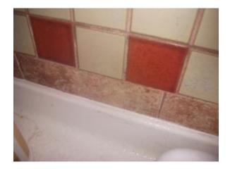
Repair: In the master shower there are areas along the lower back wall which need additional silicone. In the hall shower there are areas where additional silicone is also needed. The back splashes in the bathrooms also need silicone where they meet the counter tops.
