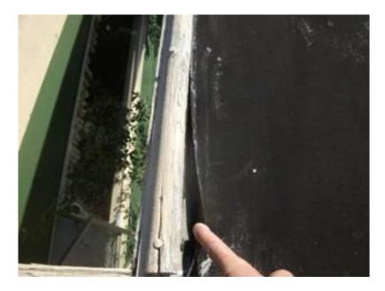
Repair: The counter flashing for the chimney has failed in many areas. This needs to be repaired by either a chimney mason or a qualified roofer. Currently with the damaged counter flashing, building framing and sheathing is exposed and is not protected by either roofing or flashing.
