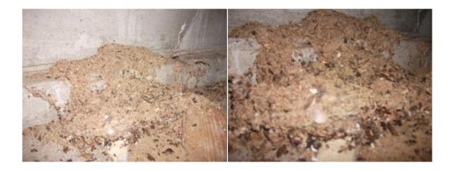
Repair: Cellulose-based debris such as wood scraps were found in crawl space (see diagram; CD). All cellulose-based debris should be removed to avoid attracting wood destroying insects.
