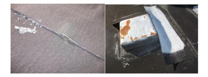
Repair: There is a skylight cut out above the entrance. The wood frame and cap have started to decay. On the walls of the frame there needs to be a counter flashing to lap over the roofing material. Currently there is none and the roof sheathing is exposed. I recommend someone qualified installs a cap to act as a counter flashing so water does not get under the roofing material.
