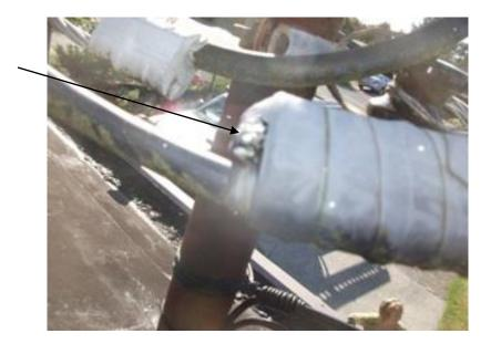
Repair: No drip loop is installed in the service entrance wires. Water may enter the service entrance conduit and equipment as a result. A qualified electrician should evaluate and repair as necessary.
