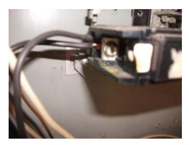
Repair: Wires in the panel are not supposed to run across the front of the panel. This wire should moved to it goes to the breaker without crossing the face of the panel.
