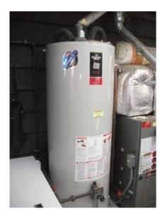
Replace: The hot water tank has failed and is leaking out of the bottom into a bucket. The hot water tank needs to be replaced by someone qualified to follow local safety codes and regulations. The above repairs are safety suggestions recommended if you were going to try and make the tank last a little longer.
